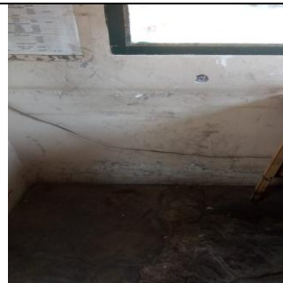
Revoque interior garita
