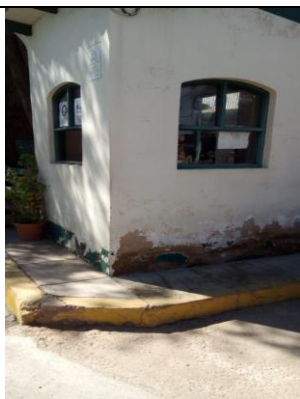
Revoque exterior garita
