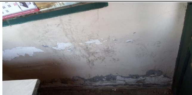
Revoque interior garita
